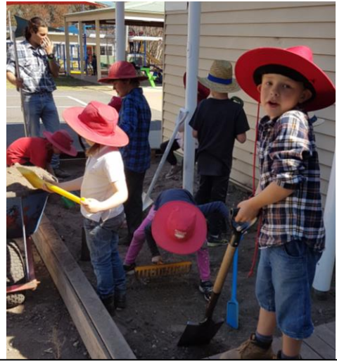
Preparing the area for our new decking to be built around the flagpoles.
